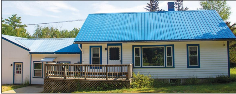
Spaulding Academy & Family Services (formerly Spaulding Youth Center) has announced the opening of a new building for its Community Based Programs staff and families. (Courtesy photo)
